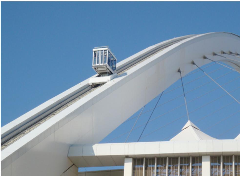
*The Moses Mabhida Stadium in Durban features a majestic steel cable-supported arch on which a funicular transports visitors 104 m in the air. Power is supplied to the funicular using conductor rails from the Single PowerLine series from Conductix-Wampfler.*
